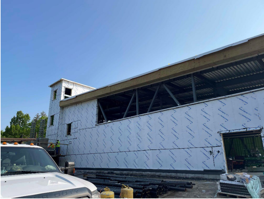
Air Vapor barrier installation
