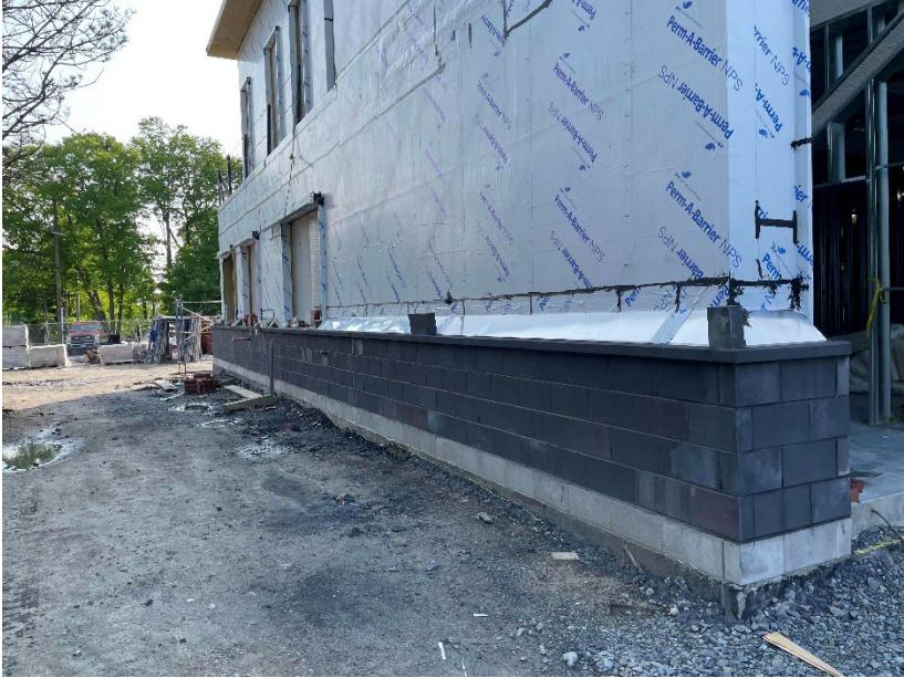
Precast stone around perimeter of building
